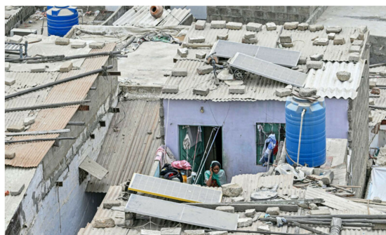
Solar panels are seen installed on rooftops in a slum in Karachi, on June 24, 2025. — AFP Fig. 3. Solar panels on rooftops.
