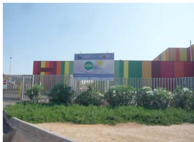
Fig. 1. ENERING+ Demonstration Site at Diego Zamora S.A. Plant (Los Camachos, Murcia)
